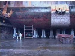
This reinforced concrete blocking line was engineered for Stolt Offshore and installed in Cape Town's Sturrock dry-dock by Wale Marine as a turn key solution. The fabrication of the 144 No cruciform shaped 200 Te SWL precast concrete units was sub-contracted to Concrete Units. This contract received the Fulton Commendation for excellence in Design in the use of concrete by The Concrete Society of Southern Africa.
