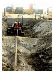
**Above** 300 Te Pipe-pulling Linear Winch for Murray and Roberts 2007 Hydraulic power unit, cylinders and controls by Hyflo. The winch operates with Amclyde Lucker grippers and is designed to allow the pulling through of spelter connections.
